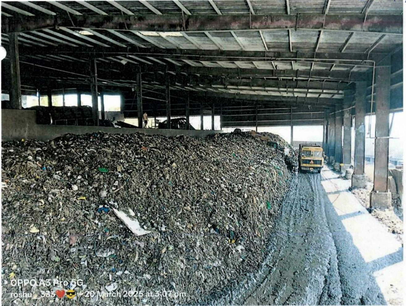
Wet waste shed No.3
